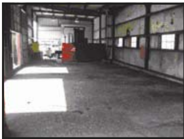
Existing Shop as of April 28, 2006
